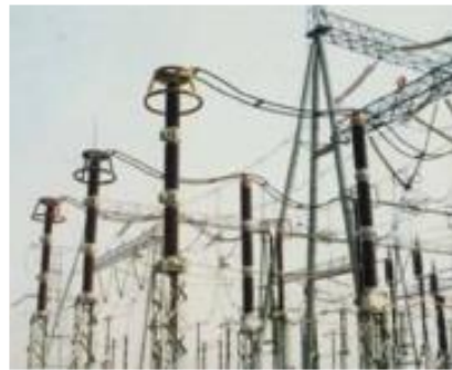
(Gambar 2.1 Lightning Arrester )
